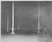
Interior view of new, epoxy-coated Tank No. 374.
